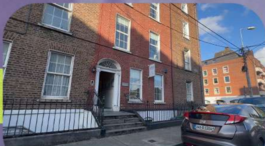
Main Building: Mallow Street (V94 K271)
